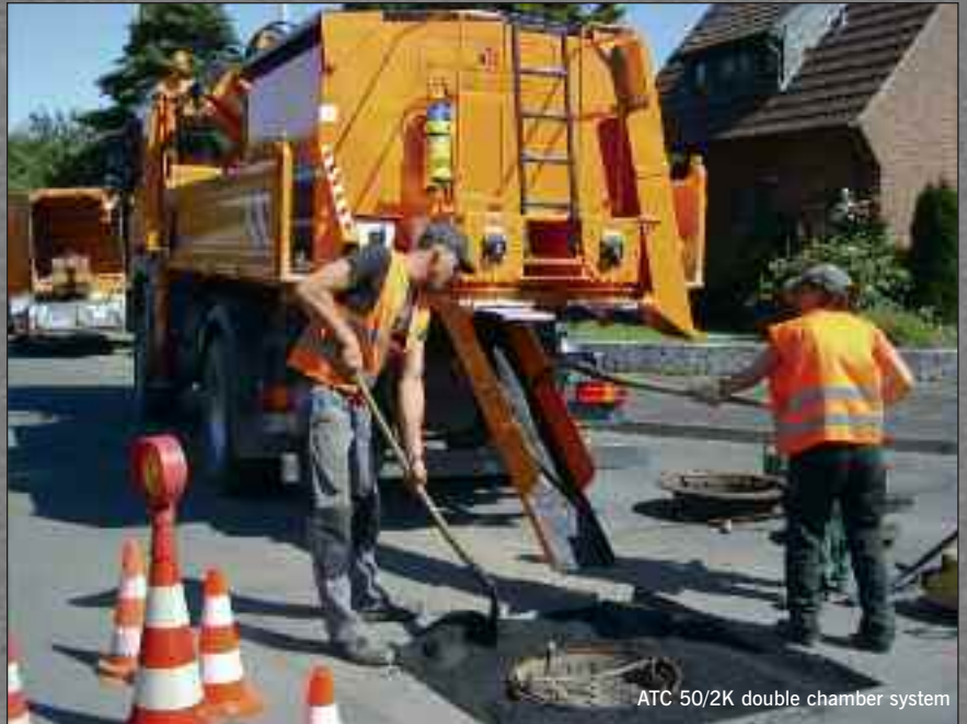
ATC 100 Single chamber system on truck
